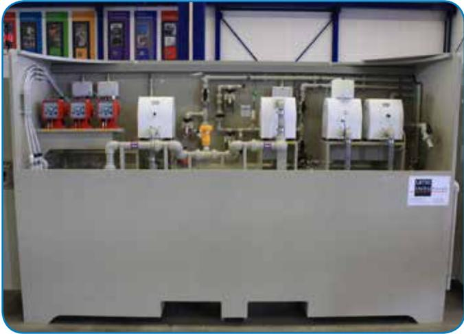
Flux-fluid systems from LBTEC INDUfinish are used to pre-treat raw steel before it is introduced to the hot-dip galvanizing process. Almatec® E-Series AODD Pumps transfer flux fluid between four distinct holding tanks during the pre-treatment process.
