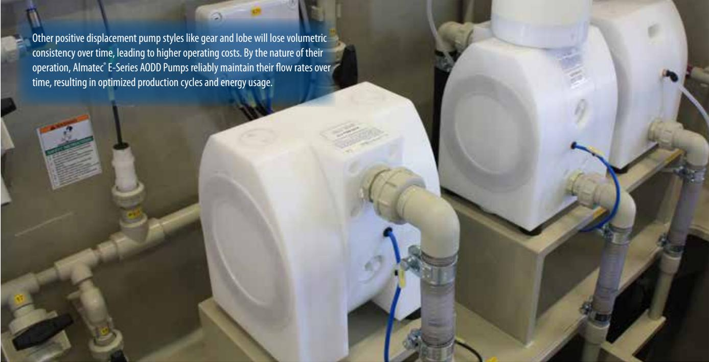
Other positive displacement pump styles like gear and lobe will lose volumetric consistency over time, leading to higher operating costs. By the nature of their operation, Almatec® E-Series AODD Pumps reliably maintain their flow rates over time, resulting in optimized production cycles and energy usage.
