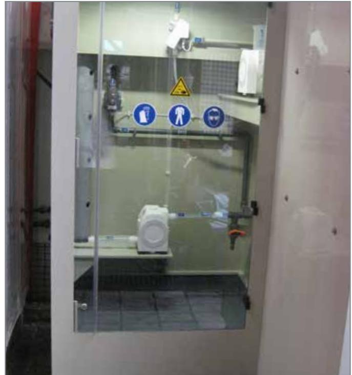
Harsh chemicals can cause compatibility concerns when used with some types of pumps. Almatec® E-Series AODD Pumps can be constructed of plastic materials that are specifically compatible with the chemicals that are being handled, which eliminates corrosion and leak fears.
