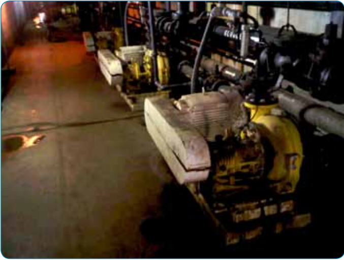
Pumps represent a large part of the facility's total investment.
