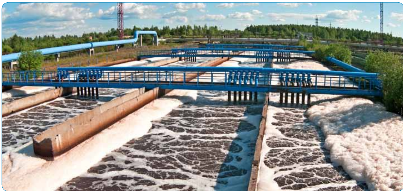
Wastewater treatment facilities utilize a variety of specialized pumping equipment along the way to providing sanitary water.
