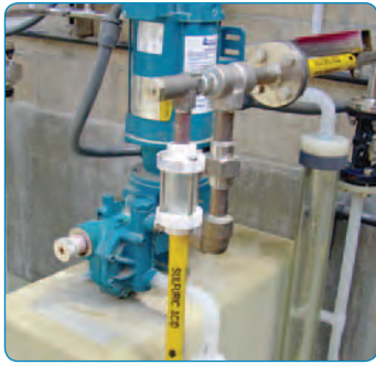
Metering pumps are reciprocating positive-displacement pumps that have the capability to inject liquids at precisely controlled and adjustable flow rates.
