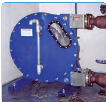
Peristaltic (hose) pumps are effective for a diverse array of applications because their operation moves products at a constant rate of displacement.
