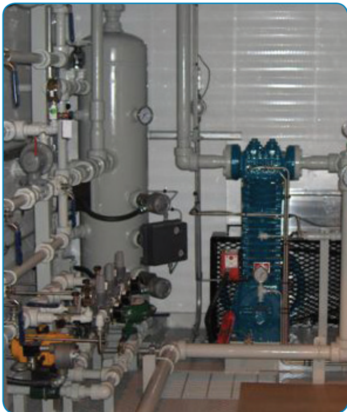
The new Quad O mandate requires that 95% of storage-tank vapor releases be contained, or either flared or reclaimed. Blackmer® Oil-Free Reciprocating Gas Compressors help ensure that that threshold is met.
