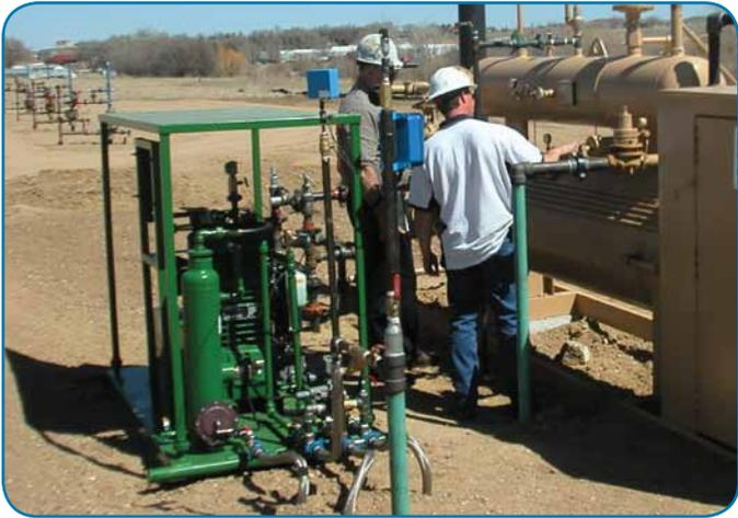
Non-lube reciprocating gas compressors help control condensate that may form inside the compressors. Blackmer compressor designs provide a means to control small amounts of condensate by collecting it in an area of the compressor called the distance-piece compartment.
