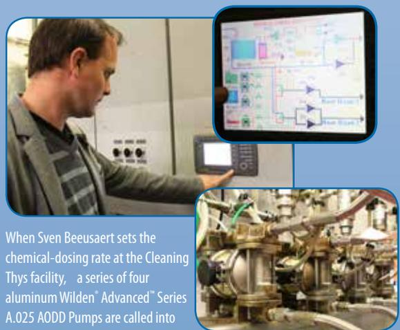
When Sven Beeusaert sets the chemical-dosing rate at the Cleaning Thys facility, a series of four aluminum Wilden® Advanced™ Series A.025 AODD Pumps are called into action.
