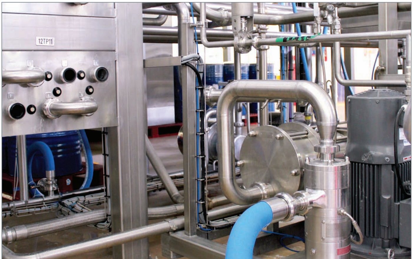
The Shiseido facility in Ormes, France, has the ability to transfer up to four tons of products per day, and thanks to their Mouvex® Eccentric Disc Pumps, the facility can expect a product recovery rate of as much as 80% or more when compared to competitive technologies.
