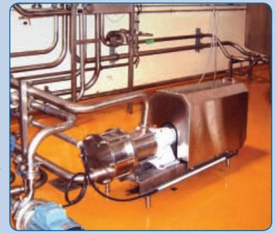
Mouvex C-Series C18i Eccentric Disc Pump.
